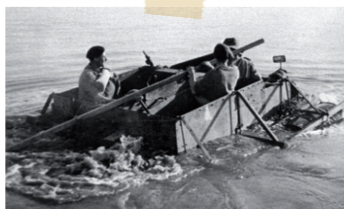
This Bren Gun Carrier belongs to the 2nd Division, and is seen negotiating the Irrawaddy River with 45 gal oil drum floats. The crossing was made after the battle of Kohima, while driving out the Japanese. (All photos Kohima Museum)
